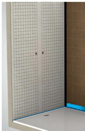
After installing the sleeves and the corner adhesive tape the sealing membrane.
