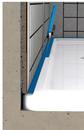
The tub attachment sealing tape on the tray is shortened to the installation height.
